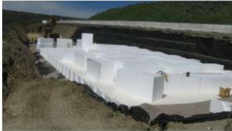
Figure 3- Geofoam used for US 50 near Montrose
