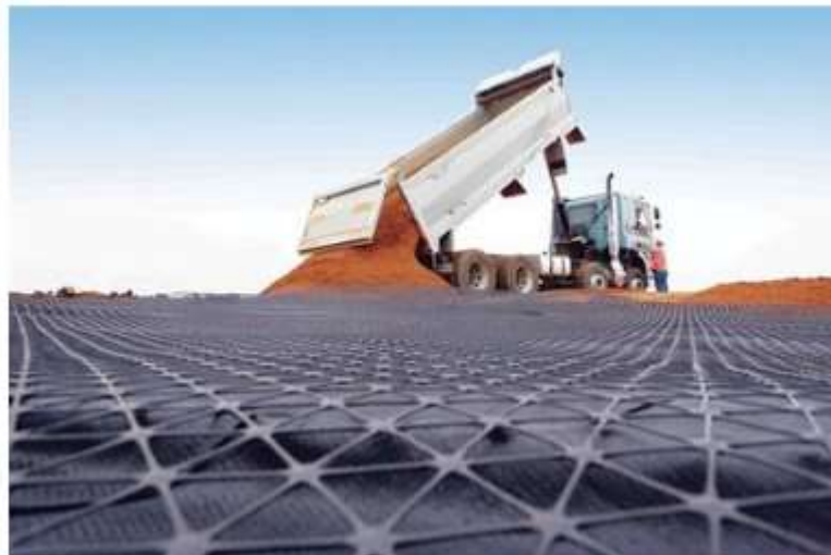
Figure 2- Geosynthetics in Road Construction on Soft Soil
